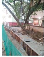
■ Pictures shot very recently show stormwater drains being constructed along the eastern flank of 1st Cross Street, Sastri Nagar.
