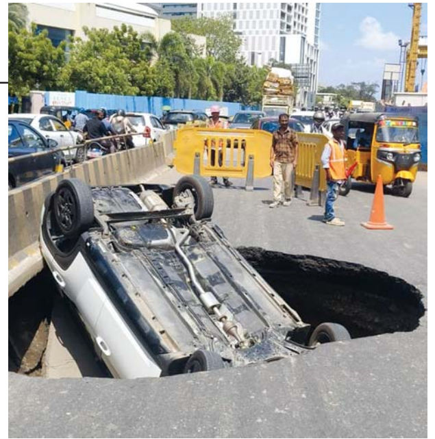
nelling operations. This collapse marks it as a recurring issue for the corridor, coming roughly a year after a similar road cave-in which occurred along the same stretch in May 2025.
